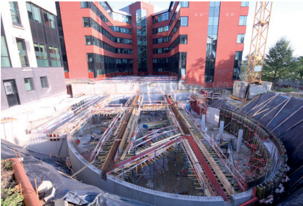
▲ Greenhouse BXL - Auditorium is taking shape
